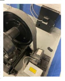
Control Type: Electric Machine Type: Traction Speed: 200 ft/min Capacity: 2,500 lbs
